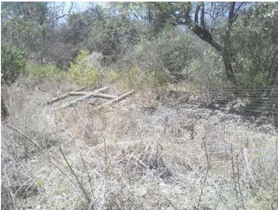
Figure 26: Part of Electric Fence Destroyed by Elephants in Meru National Park as they move to the dispersal areas
